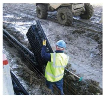
Lightweight elements, installed by one single worker.
